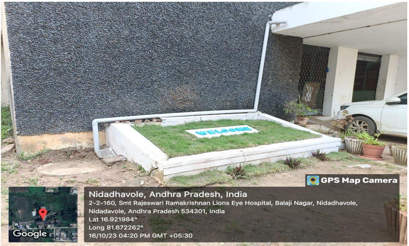
Water harvesting pit at beside of the portico
