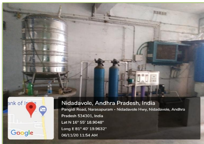
R.O. Water plant - Outlet is connected to garden
